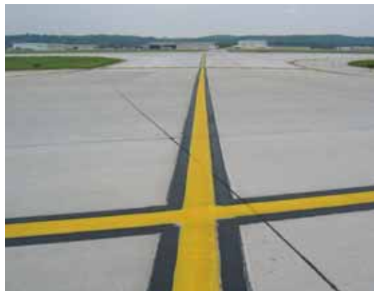
Previous Taxiway Centerline Markings
